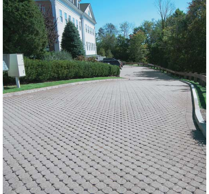
Lafayette Road Office Park - North Hampton, NH
