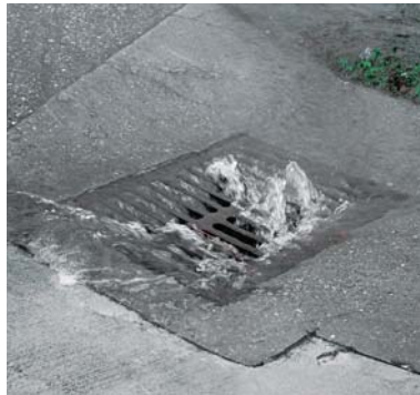
Stormwater Inlet Drain - Lake Park, FL
