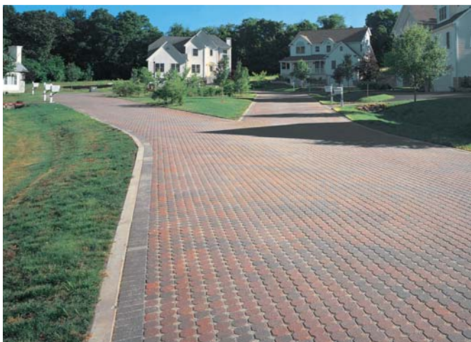
Glen Brook Green, Jordan Cove Watershed - Waterford, CT
